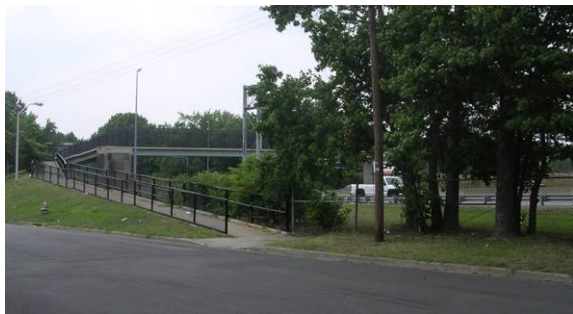
Pedestrian Overpass over I-264 – Manteo Ct at Rand St
